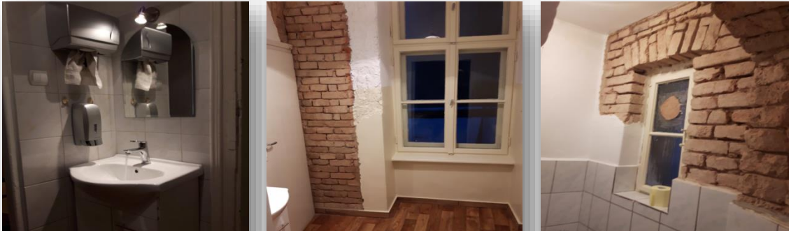
Bathroom after renovation
