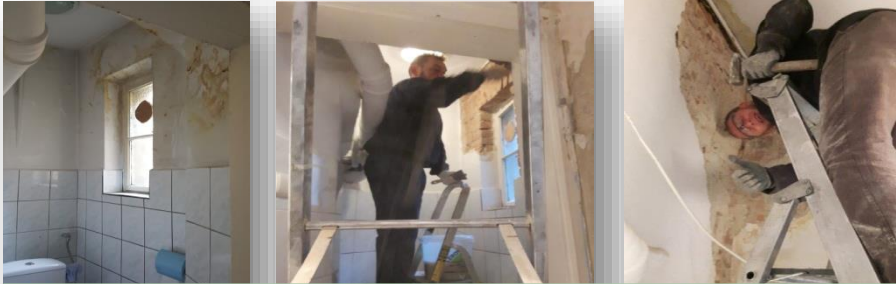
Bathroom before and during the work!
